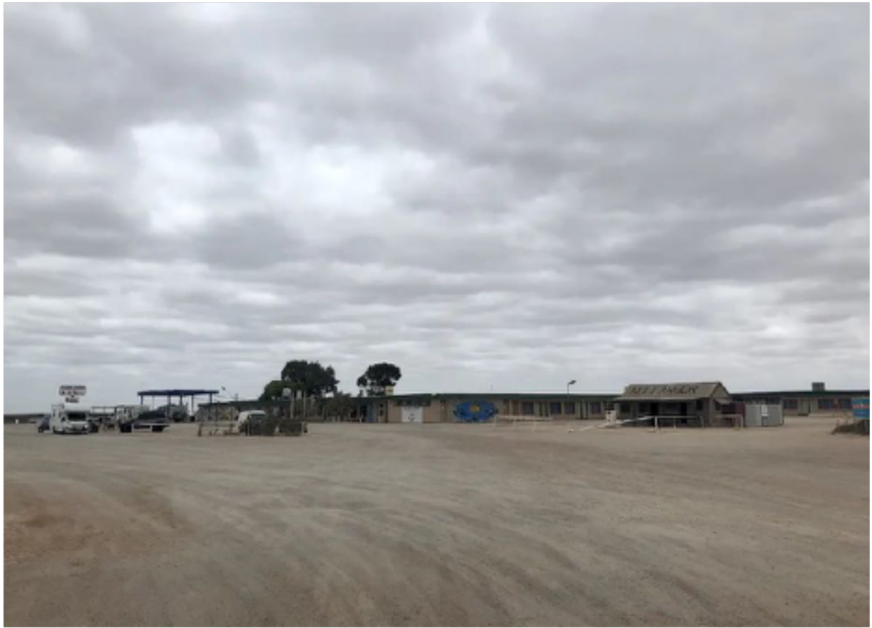
NULLARBOR ROADHOUSE. NOTE THE REPLICA OF THE ORIGINAL ROADHOUSE ON THE RIGHT. THIS WAS LOCATED JUST NORTH OF HERE AND SERVICED TRAVELLERS USING THE OLD EYRE HIGHWAY .
