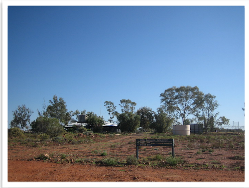
WELFORD STATION, A RARE STRUCTURE BUILT FROM RAMMED EARTH.
