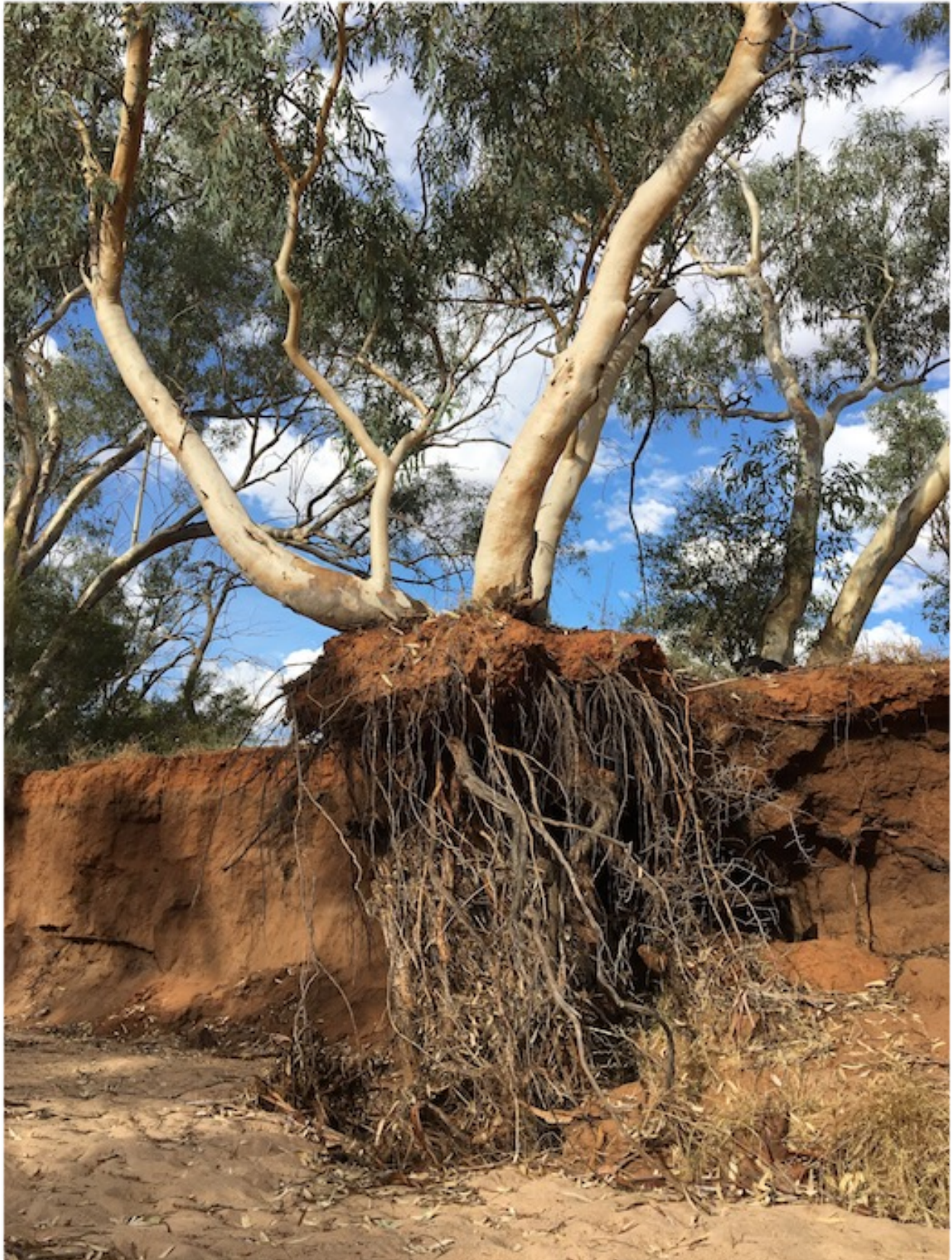
THIS GUM IS JUST HOLDING ON AFTER BEING UNDERMINED DURING A RECENT FLOOD.
