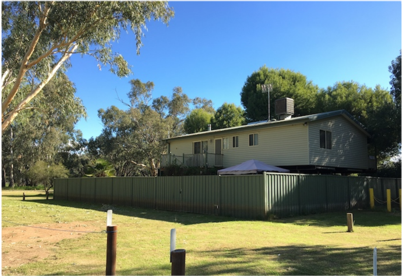
THE BROWN LINE ALONG THE BOTTOM OF THE FENCE IS ABOUT HALF A METRE HIGH - EVIDENCE OF THE RECENT FLOOD.
