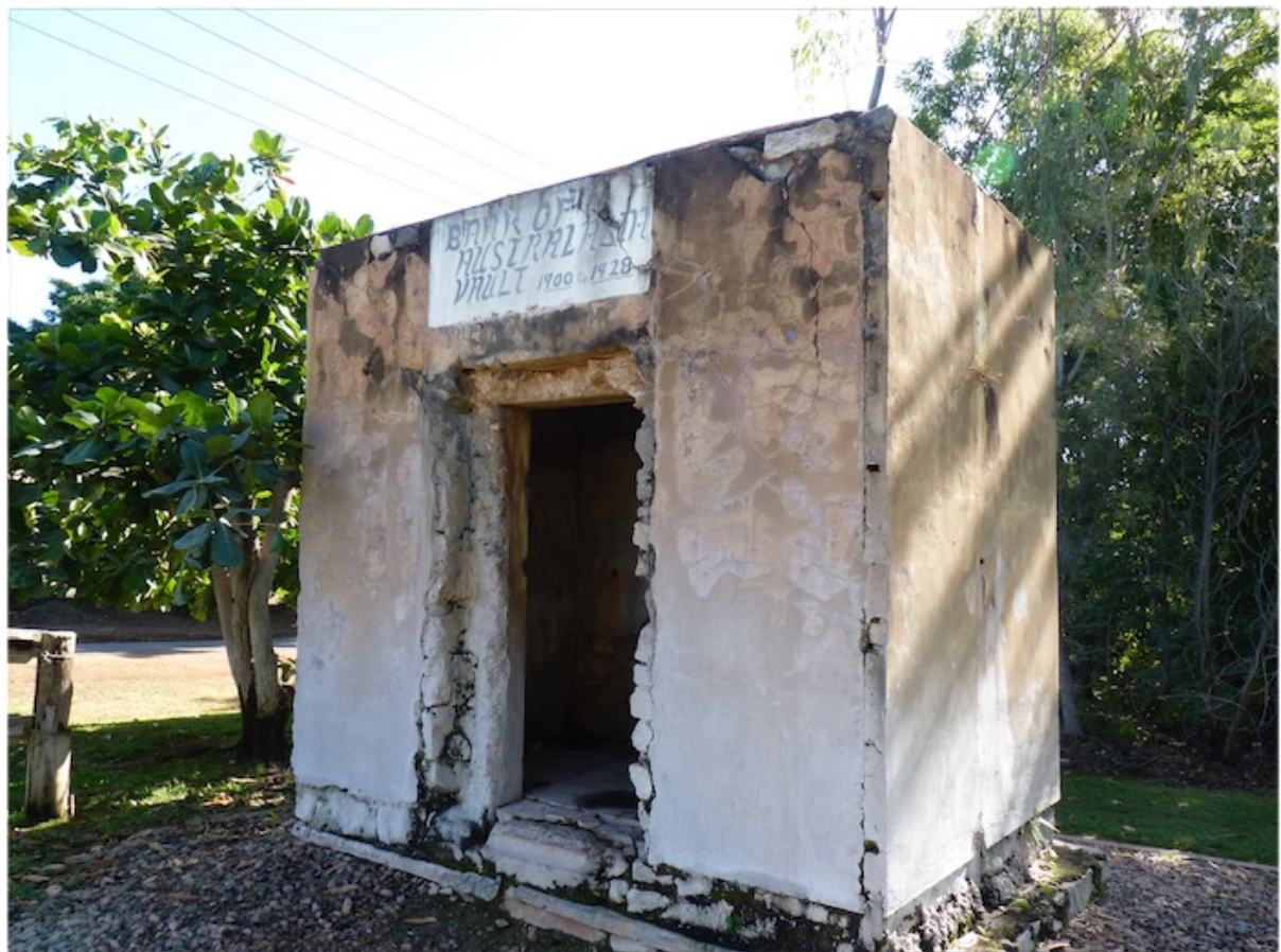
A RATHER SOLID BANK VAULT, CHILLAGOE.
